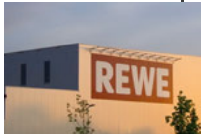
REWE-Logistikzentrum in Eitting.
